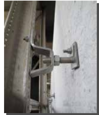
- Stainless steel brackets for connection on to steel sub channel systems
