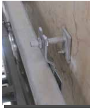
- Stainless steel brackets for connection on to steel sub channel systems
