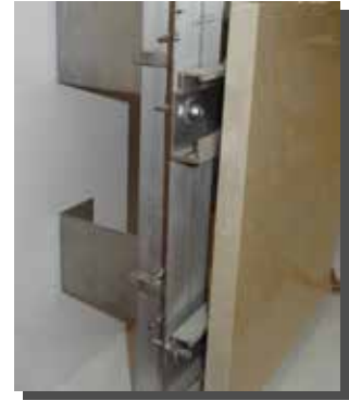
- Aluminium agraf brackets for connection into aluminium sub channel systems
