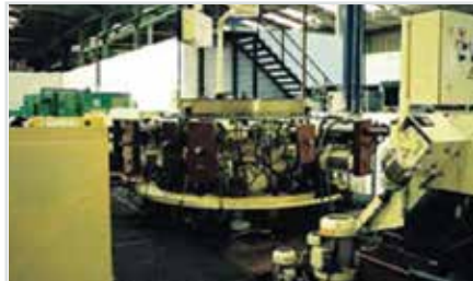
• Hydro-mat - 16 station automatic head transferer
