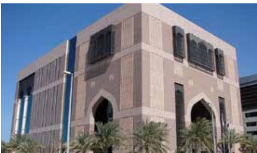
The Fund Building, Abu Dhabi
