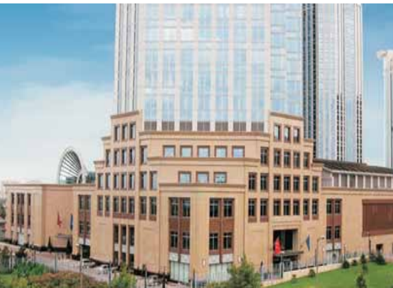
Is Bank Headquarters, Istanbul
