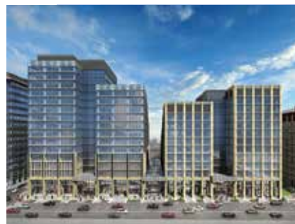
White Gardens Office Centre, Moscow
