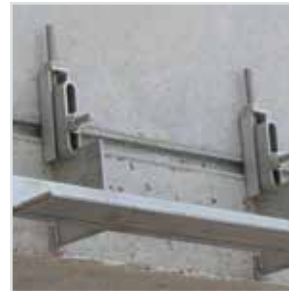
• Brickwork support systems
