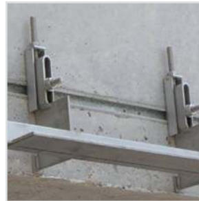
• Brickwork support systems
