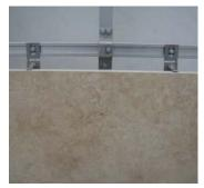
Sub channel support system provides adjustable in lateral direction. This enables quick positioning of the anchors along the horizontal channels to meet the T31 bolts fixed on the back of the stone panels.
