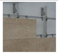
Sub channel support system designed to bear heavy loads at projection sizes exceeding 40 cm. Stone panels are installed using T31 undercut holts
