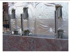
Sub channel support system designed to bear heavy loads at projection sizes exceeding 40 cm. Stone panels are installed using T31 undercut holts.
