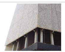
Sub channel support system provides adjustable in lateral direction. This enables quick positioning of the anchors along the horizontal channels to meet the T31 bolts fixed on the back of the stone panels.
