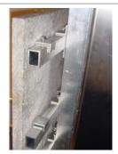
Sub channel support system provides adjustable in lateral direction. This enables quick positioning of the anchors along the horizontal channels to meet the T31 bolts fixed on the back of the stone panels.
